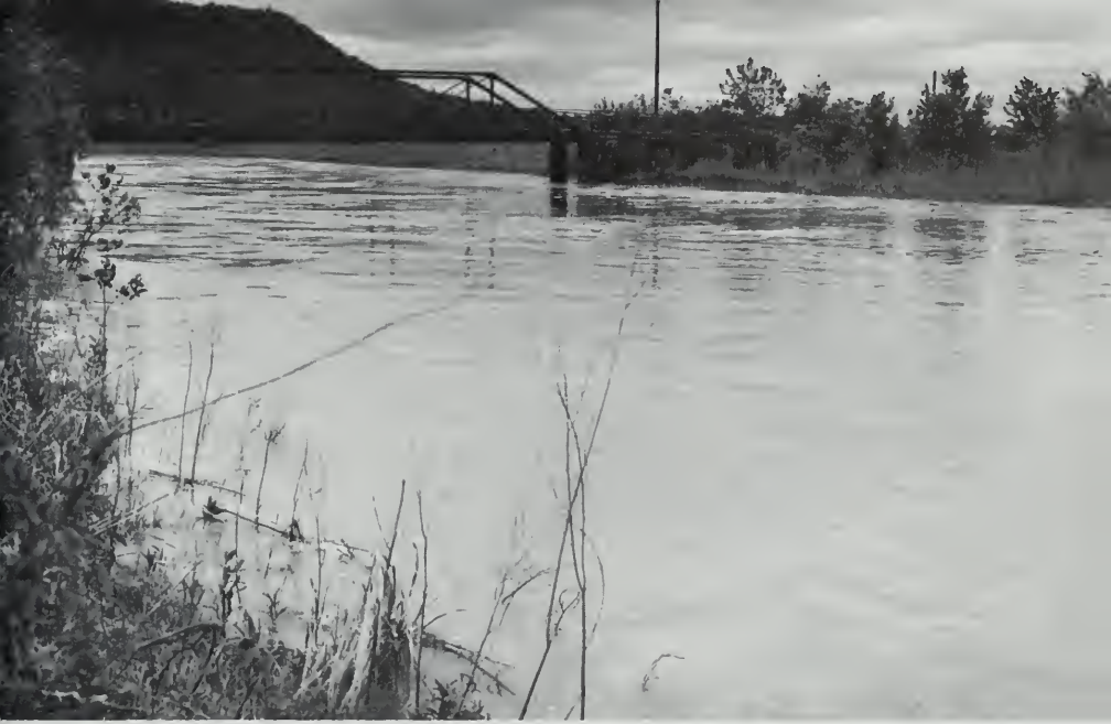
After channel improvements, Six Mile Creek flows at full capacity after a 6-inch rain.
